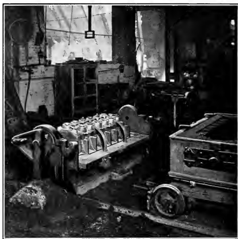
Fig. 58. Pattern Mounted on Roll-Over Jolt Machine.
